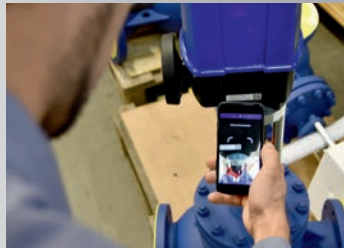
On-site scanning of the ARI-ID with a smartphone
